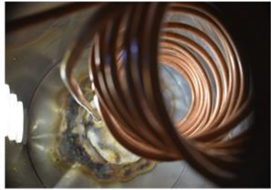
FIGURE 5 | The heat exchanger (coil exchanger).
