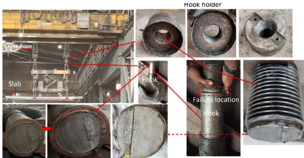
FIGURE 2 | Visual examination of the EOT crane hook showing failure at a thread groove region.
